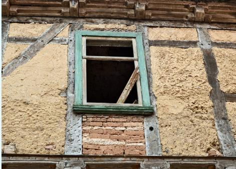
**Top:** This half-timbered building in Wettin, Saxony-Anhalt (Germany), shows several forms of surface preparation for a better adhesion of the plaster. Besides the plaster having been incised with various grooves, the panel beams were also hewn with a hatchet (photo: F. Knoll 2016).
