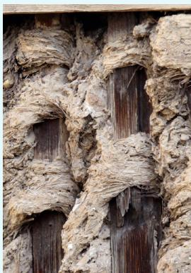
**Top left:** Weathered »Lehmwickel« (»dutch biscuits«) at a decayed half-timbered house in Halle (Saale), Saxony-Anhalt (Germany; photo: F. Knoll 2017).
