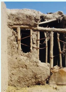
**Right:** Timber frame with earth infill, abandoned »sintch« building, Khiva, Xorazm Region (Uzbekistan; Cooke 2010, 64 Fig. 39).
