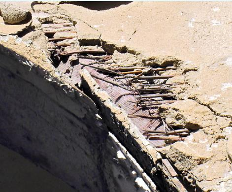
Reed used to achieve a better plaster adhesion in a half-timbered building in Quedlinburg, Saxony-Anhalt (Germany; photo: M. Pastor Quiles 2017).
