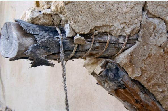
Cords twined/twisted around a wooden building element for an improved adhesion of the plaster. Aspe, Alicante (Spain; photo: M. Pastor Quiles 2015).
