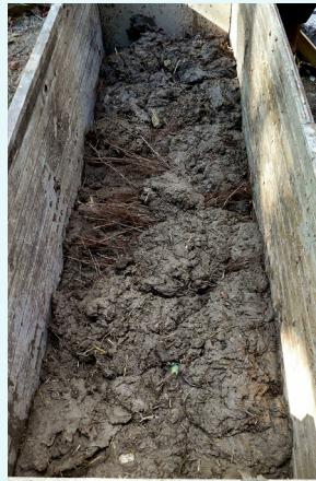
Lattes, Hérault (France), experimental workshop. Constructing a wall by packing cob layers into the wooden frame, separated by branches of heather (photos: C.-A. de Chazelles 2010).
